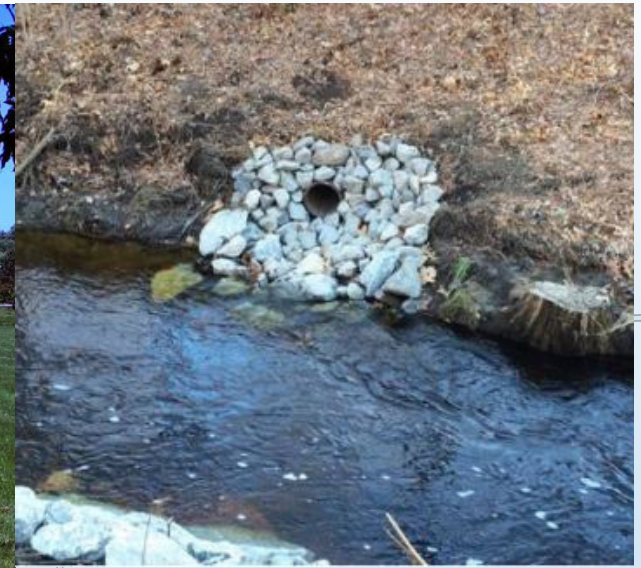
Erosion retrofit strategy for stormwater outfall Source: Wellesley, MA
